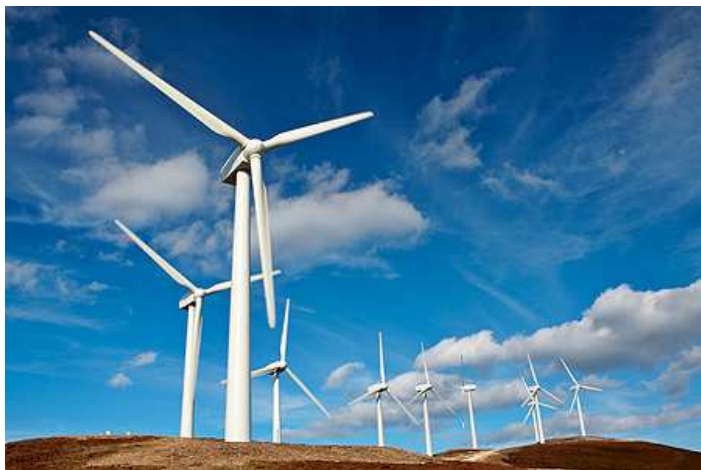
Typical Wind Farm
