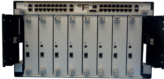
the Aurora HPC 20-22 chassis mounted in the G-Station
